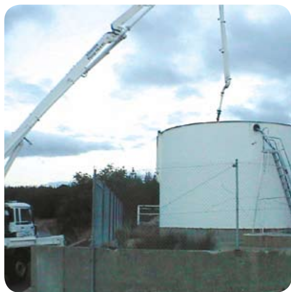
Encapsulation of the mercury sludge.
