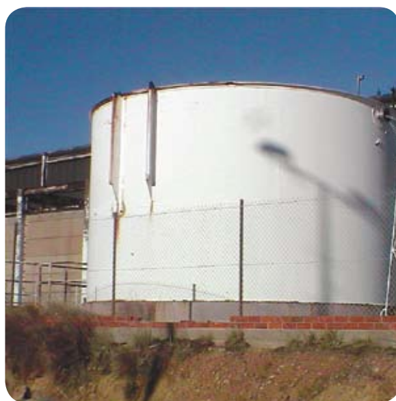
Mercury sludge tank.
