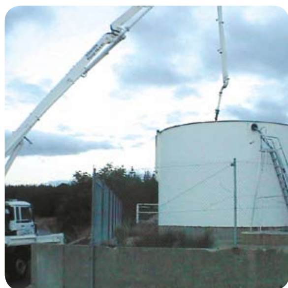
Encapsulation of the mercury sludge.
