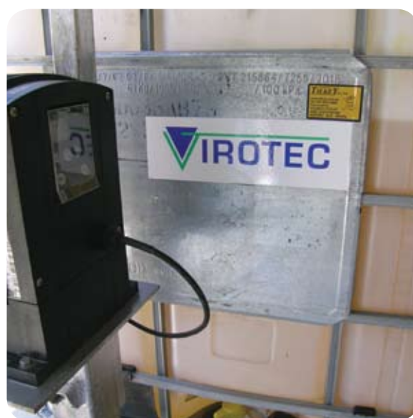
The dosing point for ViroPhos™ Reagent B.
