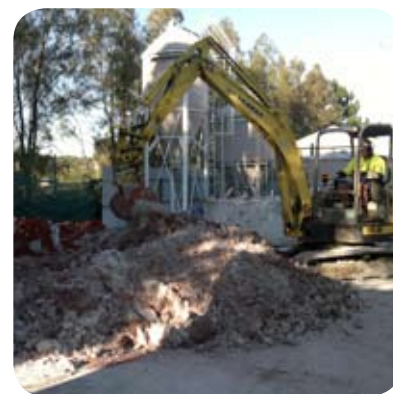
Mixing the ElectroBind™ Reagent with the sludge waste
