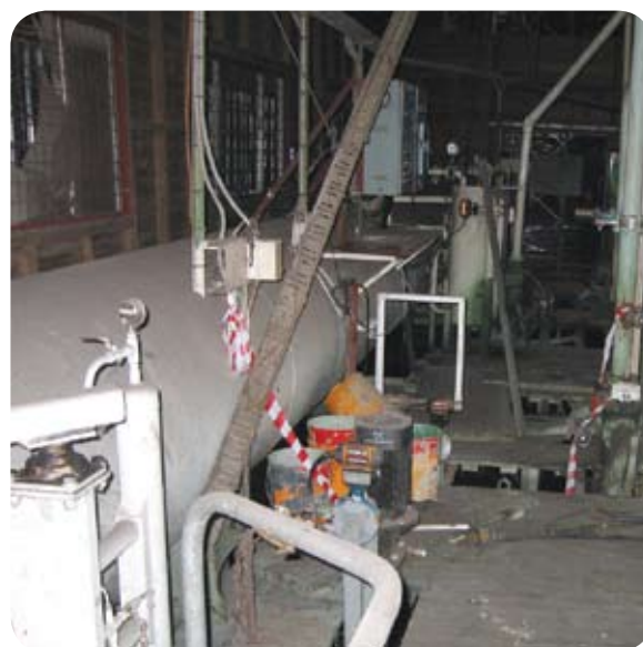
Exposed internal moats contaminated by CCA where ViroFlow™ Technology treatment was applied.
