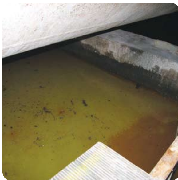
Suspended ViroBond™ reagent particles that bound the heavy metals have settled to the bottom following treatment.
