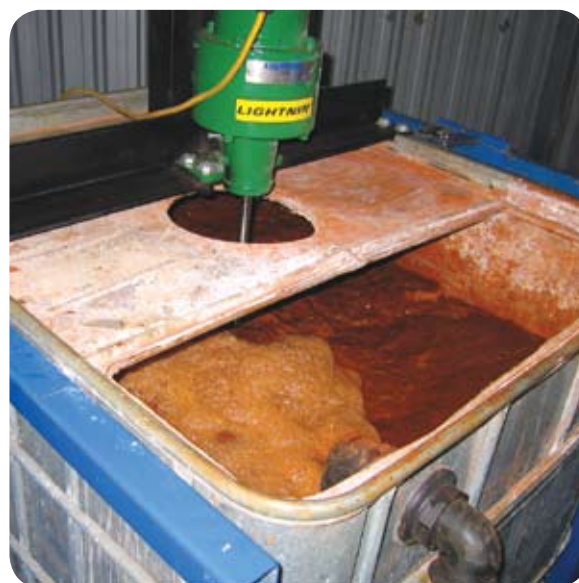
Virotec's mobile ViroFlow™ Technology Mixing and Dosing Plant being used to treat the moats.
