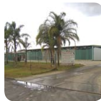
The Hyne Timber preservation facility being decommissioned.
