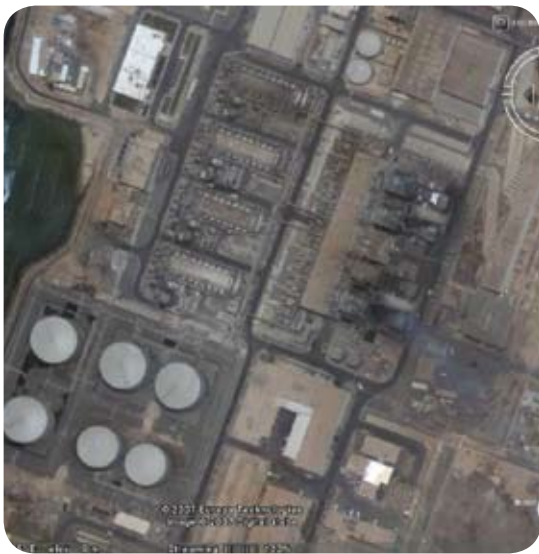
Aerial view of the salination plant in Jeddah
