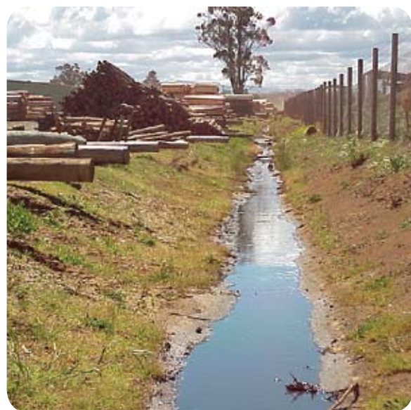
The stormwater drain leading from the timber storage area to leachate pond.
