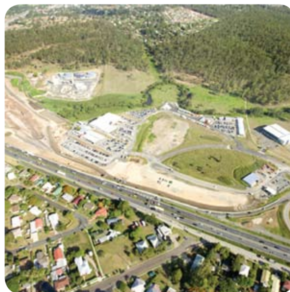
An aerial view of the Dinmore to Goodna motorway upgrade
