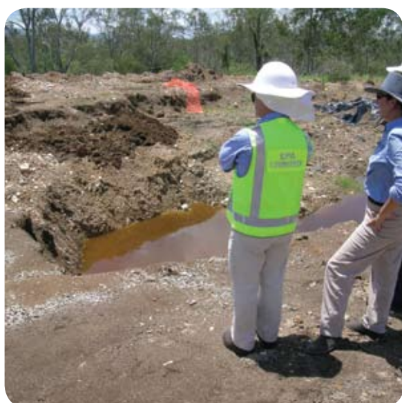
Queensland EPA was present during excavation of contaminated soil
