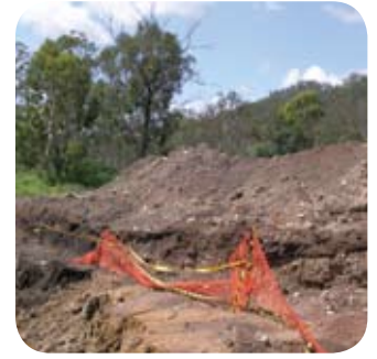
Contaminated stock pile of soil prior to treatment
