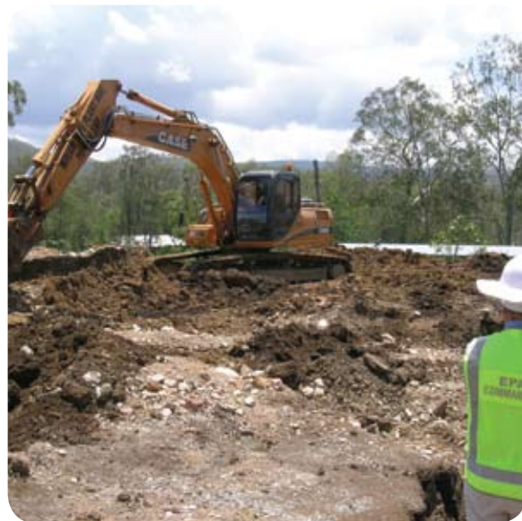
Contaminated soil being excavated so treatment can commence
