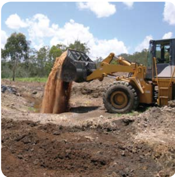
Excavation of contaminated soil
