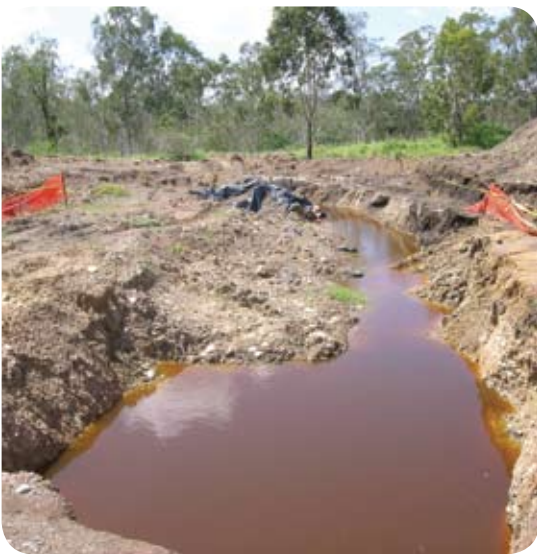
Excavated area before treatment with ViroFlow™ Technology
