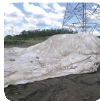
Stock pile of contaminated soil prior to treatment at external facility
