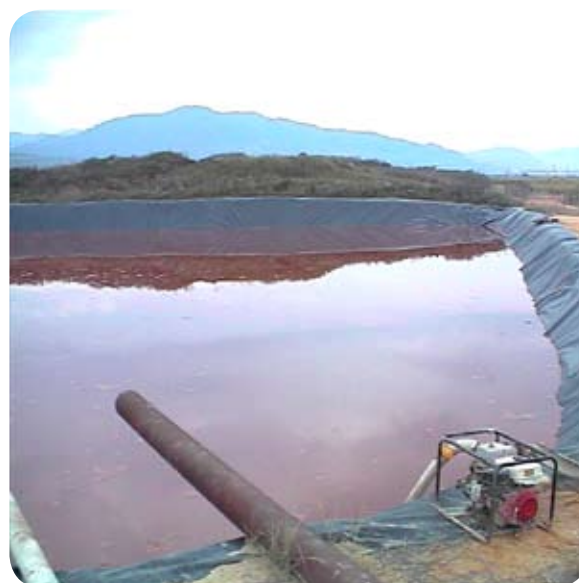
This pond was constructed to conduct the Acid B Extra™ reagent AMD treatments in Baia Mare. The pond was lined with geosynthetic liners and contained 2 ML of water.
