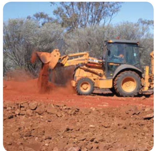
ViroMine™ Technology is alleviating past issues with in-situ immobilisation of metals and neutralisation of acid mine drainage.
