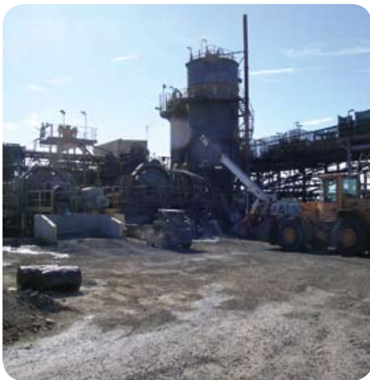
Fox Resources Processing Plant
