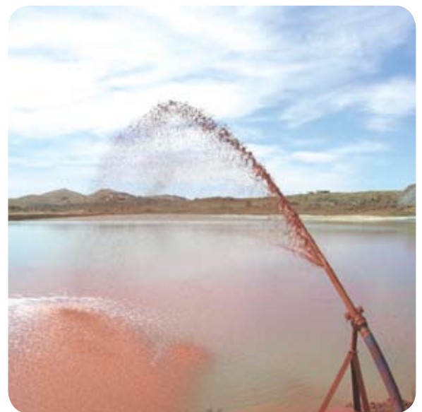
Acid B™ reagent slurry being applied to the tailings dam.
