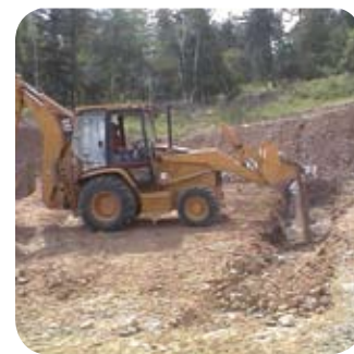
Preparing the Permeable Reactive Barrier Trench.
