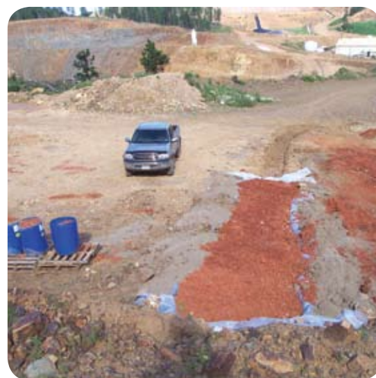
Preparing the Permeable Reactive Barrier Trench.
