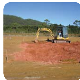
The Terra B™ reagent was spread and mixed into the tailings using an excavator.
