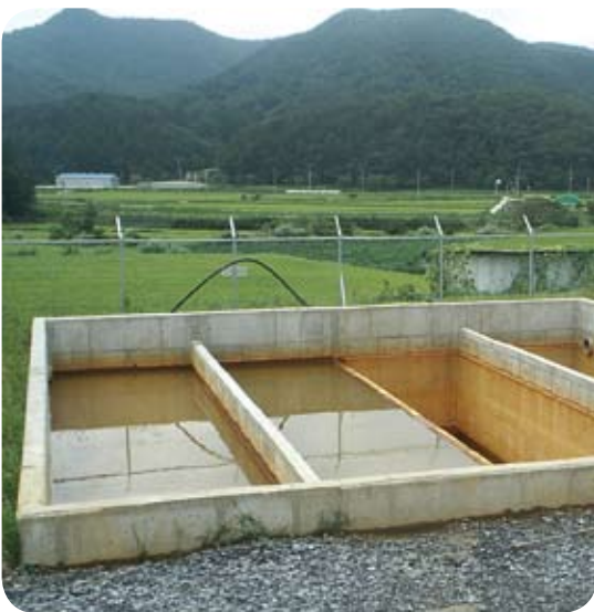
Filtration systems utilising ViroMine™ Technology
