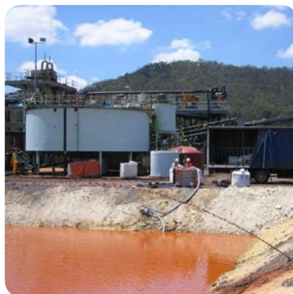
The Virotec operations team pumping contaminated holding dam water to the treatment facility (rear)
