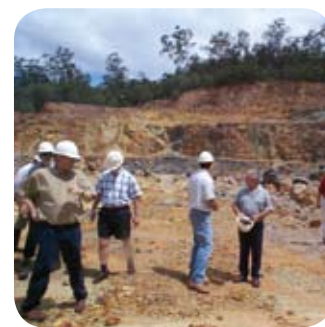
Treated water from the Tailings Dam being independently tested by government officers and released into local catchment.
