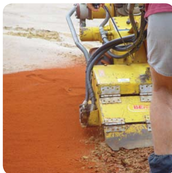
Mixing the Terra B™ reagent with the tailings.
