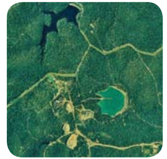
An aerial shot of the Tailings Dam.
