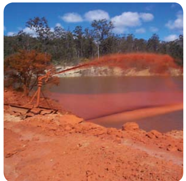
Acid B™ reagent was applied as a slurry mixture and sprayed onto the surface of the dam.
