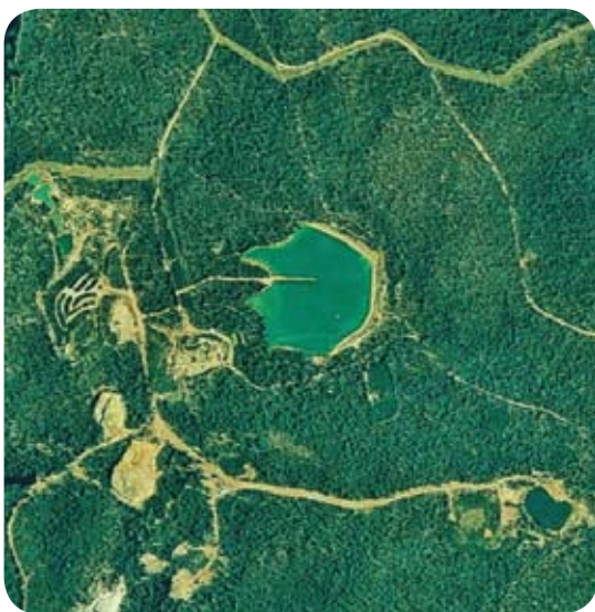
The Mt Carrington Tailings Dam
