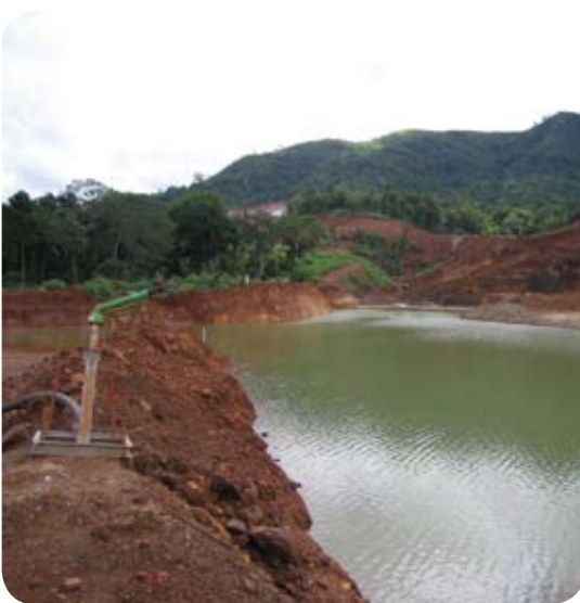
The Khanong attenuation pond
