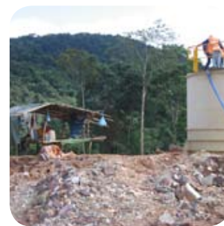
A mixing tank at Sepon Gold Mine.
