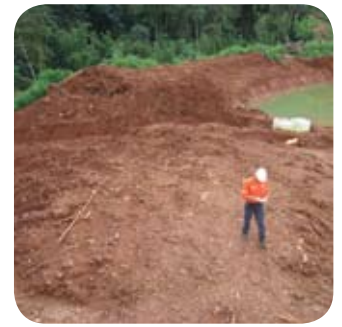
The spillway for Khanong AMD attenuation pond
