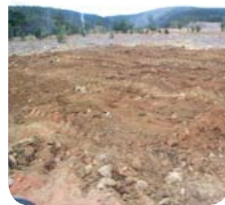
The fully remediated Zn-enriched tailings plot at Rossarden prior to revegetation with poa grass seedlings.
