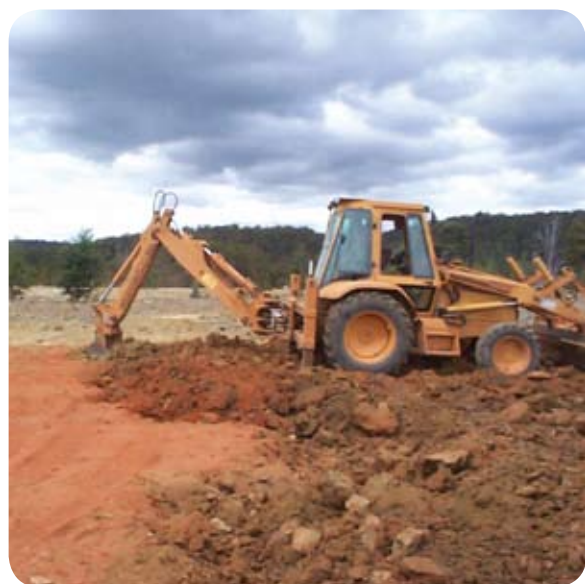
Terra B™ reagent being mixed into the zinc-enriched tailings with the backhoe.
