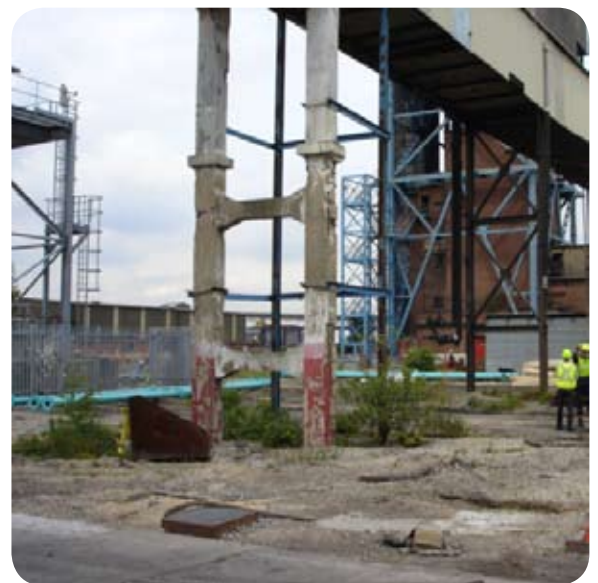
Site of ViroMine Technology treatment system at UK Coal's Maltby Colliery site
