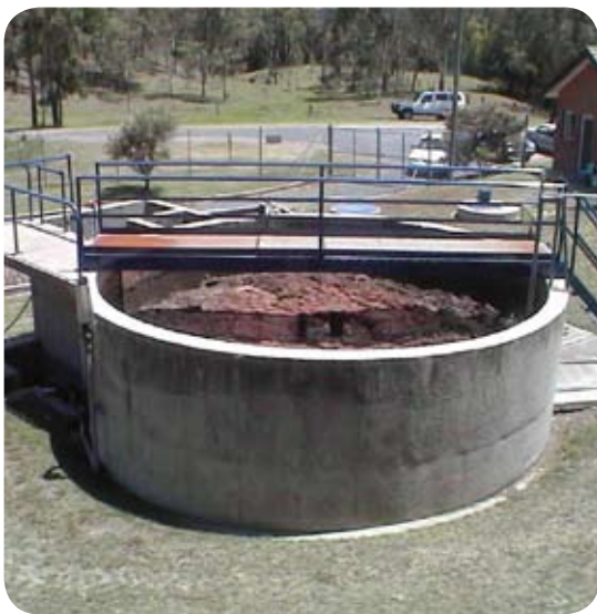
An overview of the Sewage Treatment Plant.
