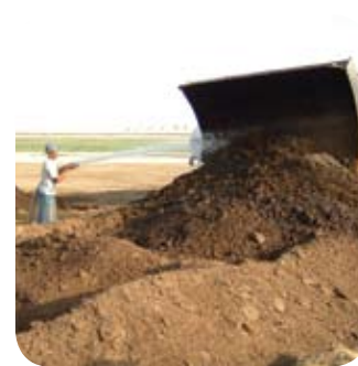
Mixing of the ViroBlend™ reagent into the waste product
