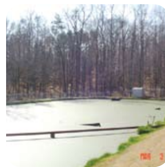
The facility has two lagoons each with an approximate capacity of 1 ML.
