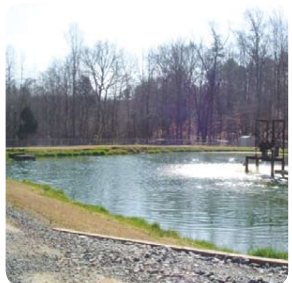
Lagoon #1 after treatment using ViroSewage™ Technology
