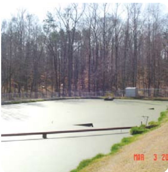
Shandon Lagoon prior to treatment
