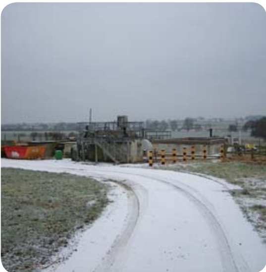
The entry road to Kirk Smeaton Sewage Treatment Plant in West Riding, Yorkshire
