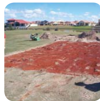
Mixing the ViroBind reagent into the sand.
