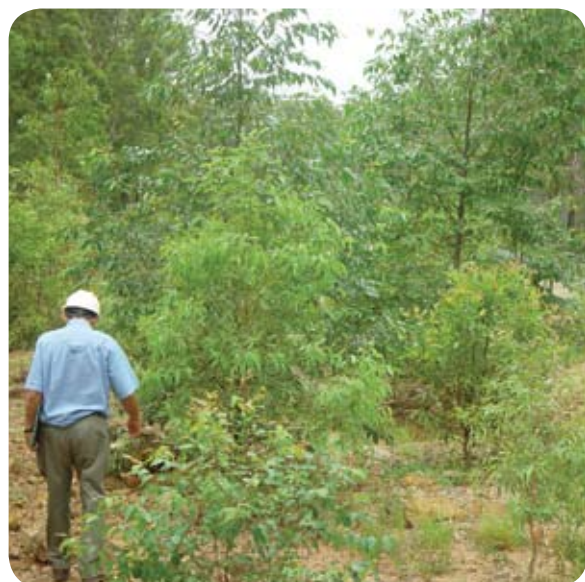
Haul road after treatment.
