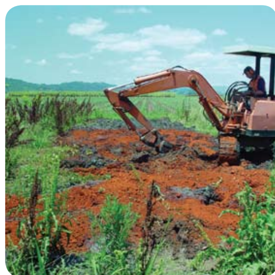
ViroBind™ reagent being mixed with the Acid Sulphate Soil to neutralise acidity and promote crop growth.
