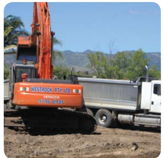
Treated soil being transferred offsite to landfill.
