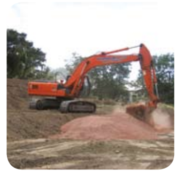
Stockpile of ViroBind™ reagent prior to blending with contaminated soil.
