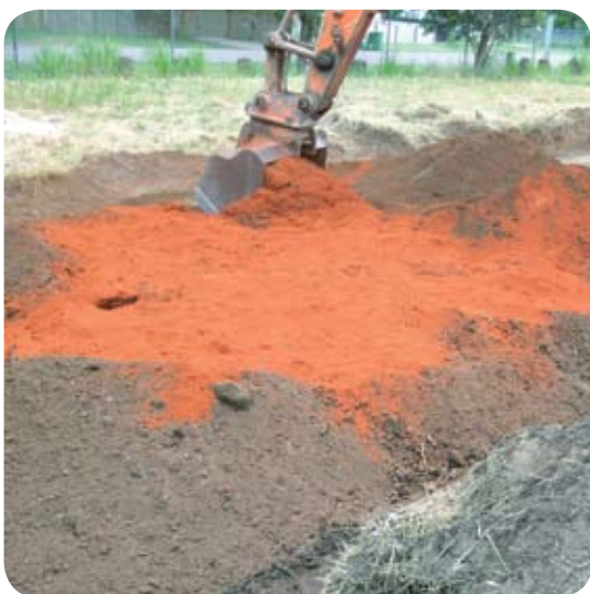
ViroBind™ reagent being mixed into the contaminated soil.
