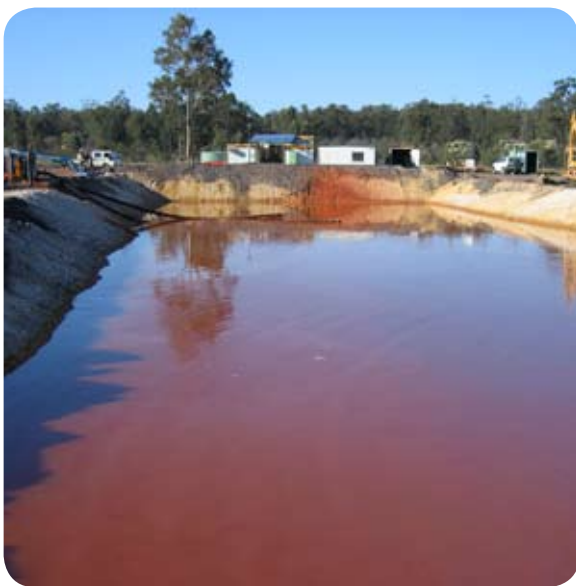
The holding dam which was treated by ViroMine™ Technology at a large coal mine in New South Wales, Australia
