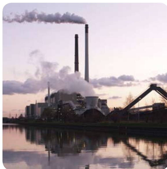
A coal fuelled power station
