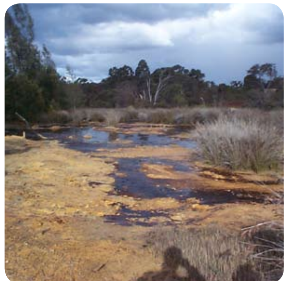
Dam seepage at Aberdare East Colliery
