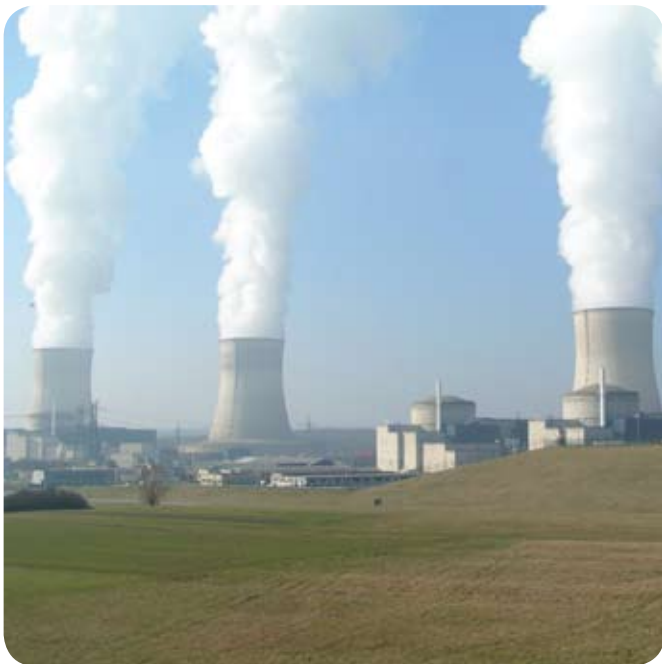
View of Cooling Towers.
