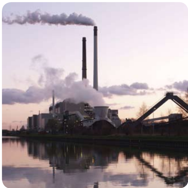
A coal-fired electrical plant
