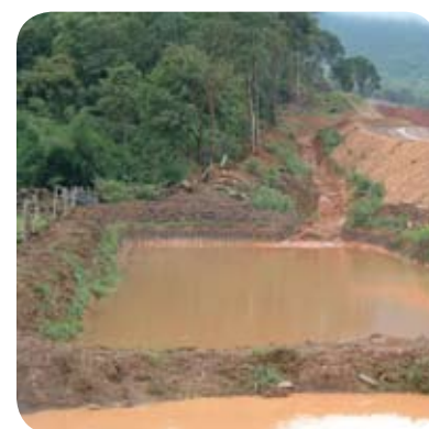
Example of a drainage gallery parallel to a road (centre rear) and stormwater attenuation dam (centre)
