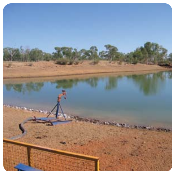
Dam stormwater quality after treatment
