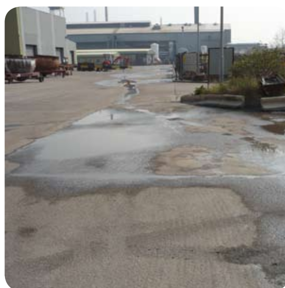
Open areas of impermeable roadways and concrete pads
