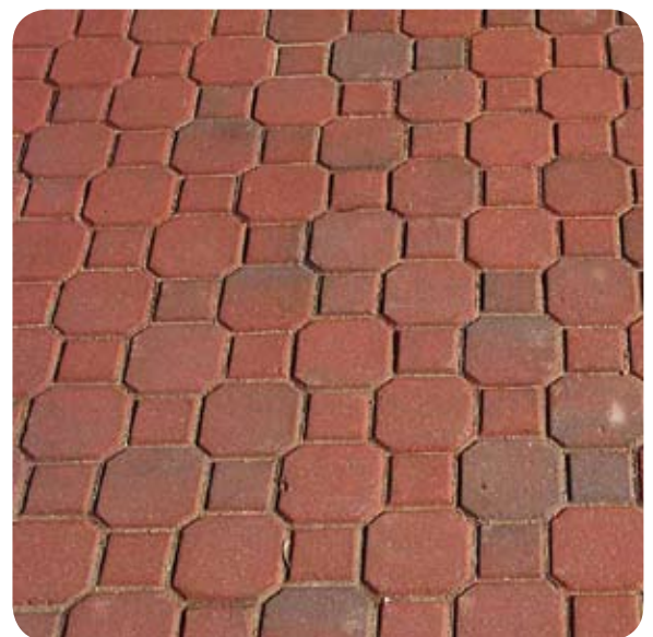
Example of permeable pavers
