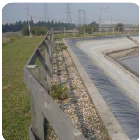
Stormwater is held in this PVC-lined holding dam prior to treatment and discharge
