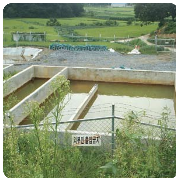
The over-under baffle treatment system, with discharge point in distance (rear)
