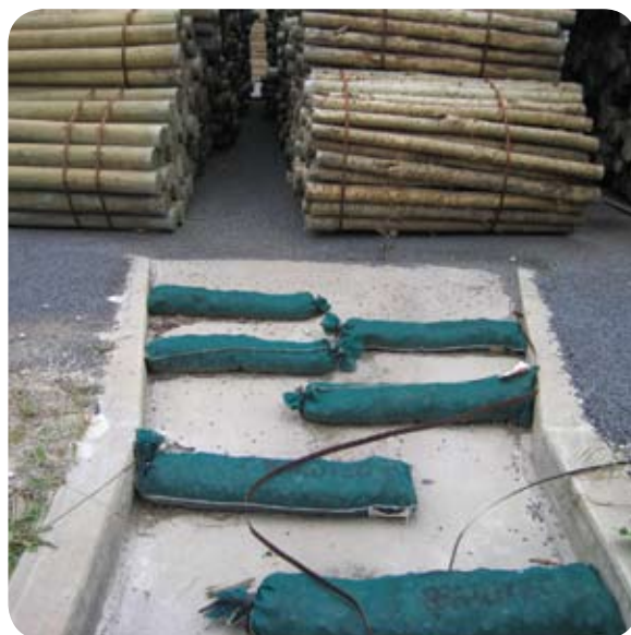
Geotextile filter bags placed in CCA-contaminated stormwater drains
