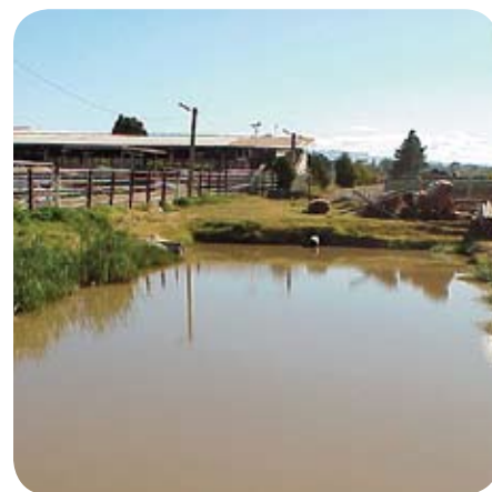
A leachate pond before treatment
