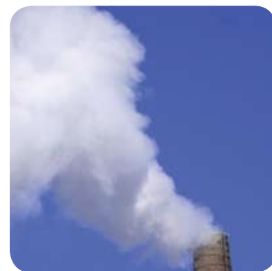
Sewage treatment plants, industrial plants, paper pulp mills, tanneries and facilities like piggeries are increasingly being subjected to odour production limits.
