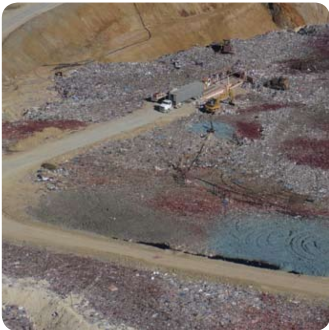
Woodlawn Bio-reactor, NSW
