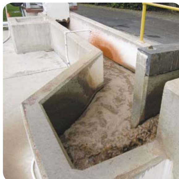
Example of dosing ViroFilter™ Technology as slurry at location 2 in Figure 10, into the Return Activated Sludge (“RAS”) line at Brisbane Water, Australia
