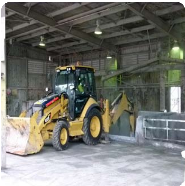
Contaminated demolition waste loaded into treatment pits ready for ViroFlow™ Technology treatment at Virotec's Queensland facility.
