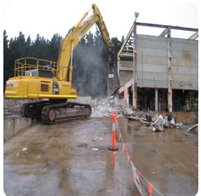
Demolition of a building's superstructure using a 40 tonne excavator.
