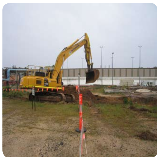
Excavating contaminated soil post superstructure demolition.
