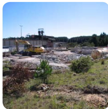
Immediate post-building demolition phase prior to concrete slab and tank removal.
