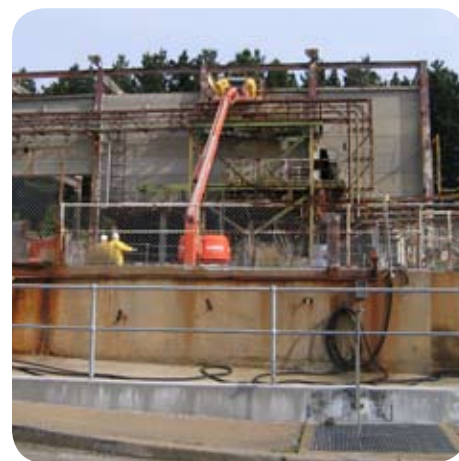
Asbestos sheet removal prior to primary superstructure demolition.
