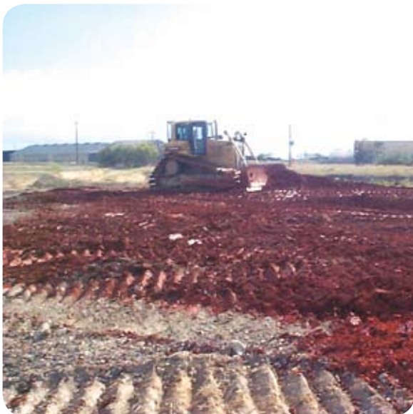
Application of ViroBind™ reagent at Port Gladstone
