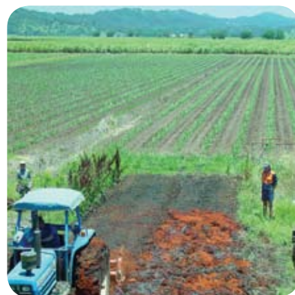
Mixing ViroBind™ reagent into ASS at a sugar cane farm in northern NSW
