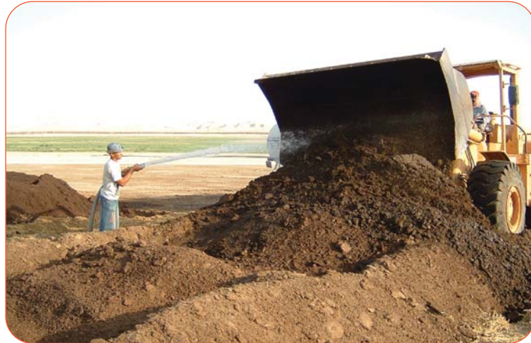
Figure 3 - Mixing of the ViroBlend™ reagent into the waste product
