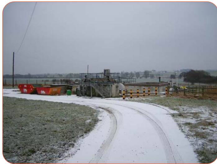
Figure 2: The entry road to Kirk Smeaton STP in West Riding, Yorkshire
